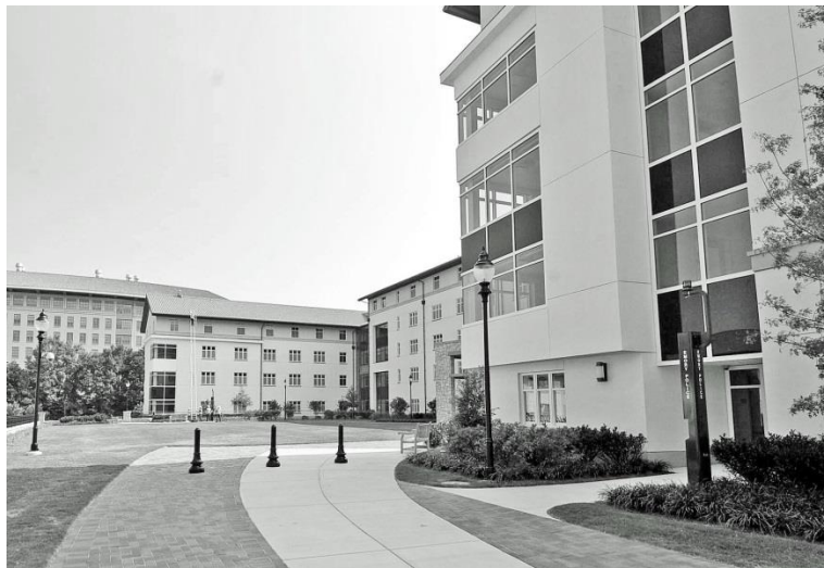
Figure 4 – Turman Hall sand media filter system plaza over a parking garage at Emory University, Atlanta, GA
